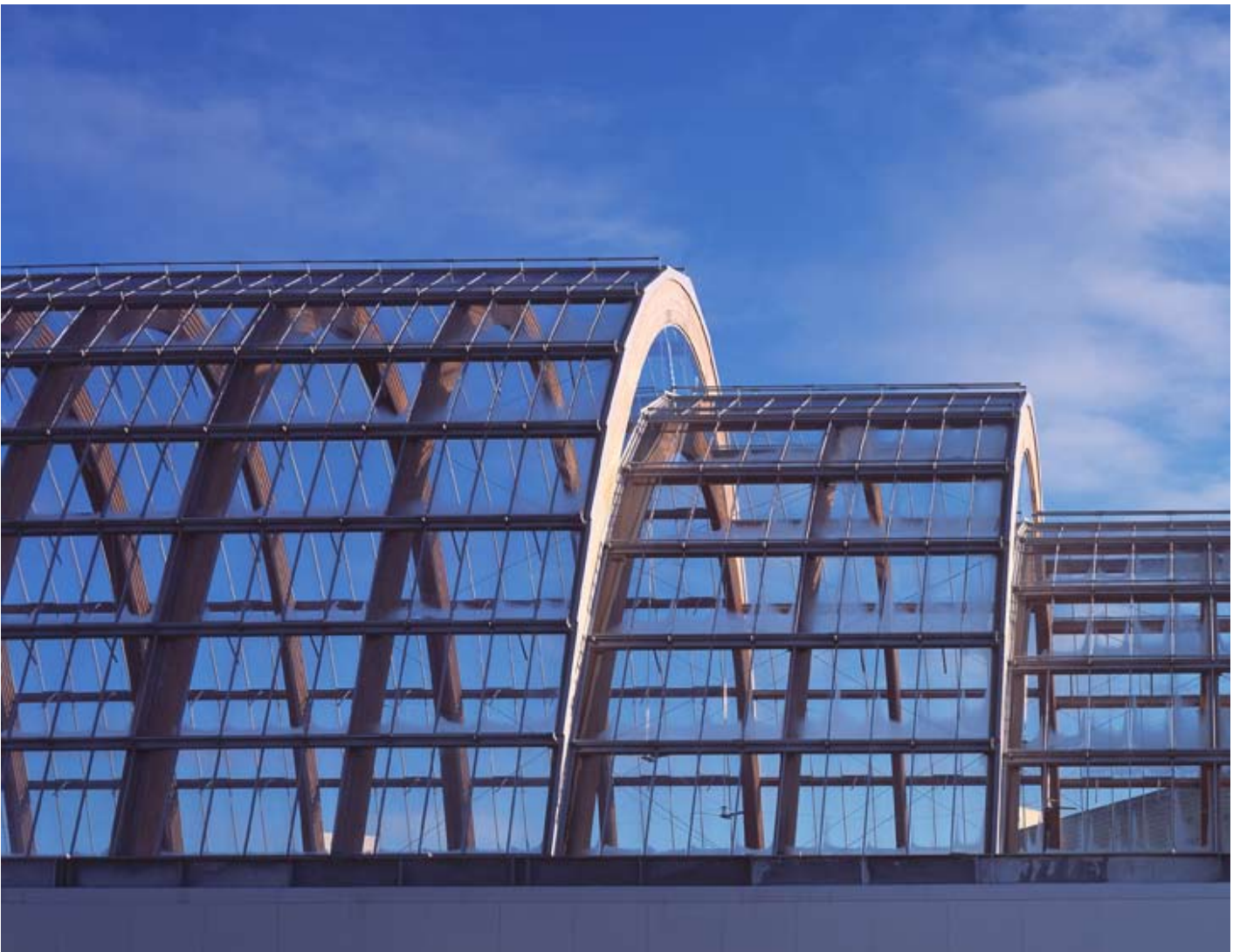
Above: Winter Garden roof profile with parabolic structure in larch
