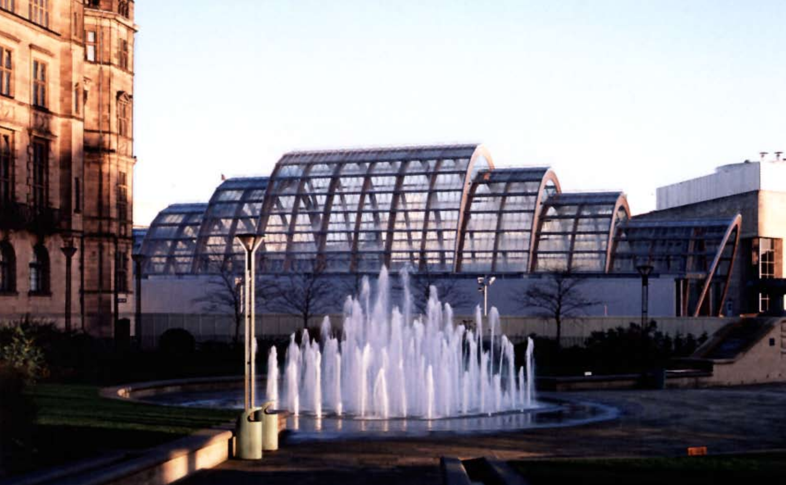
Left: 70 metre long Winter Garden seen across the Peace Gardens Below: canopy over Peace Gardens entrance
